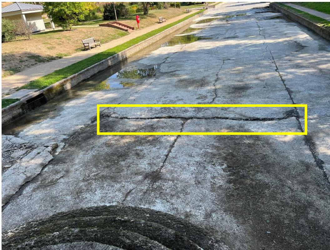
Plate 1 – View from upstream end of pond showing cracking and voided area A15.
